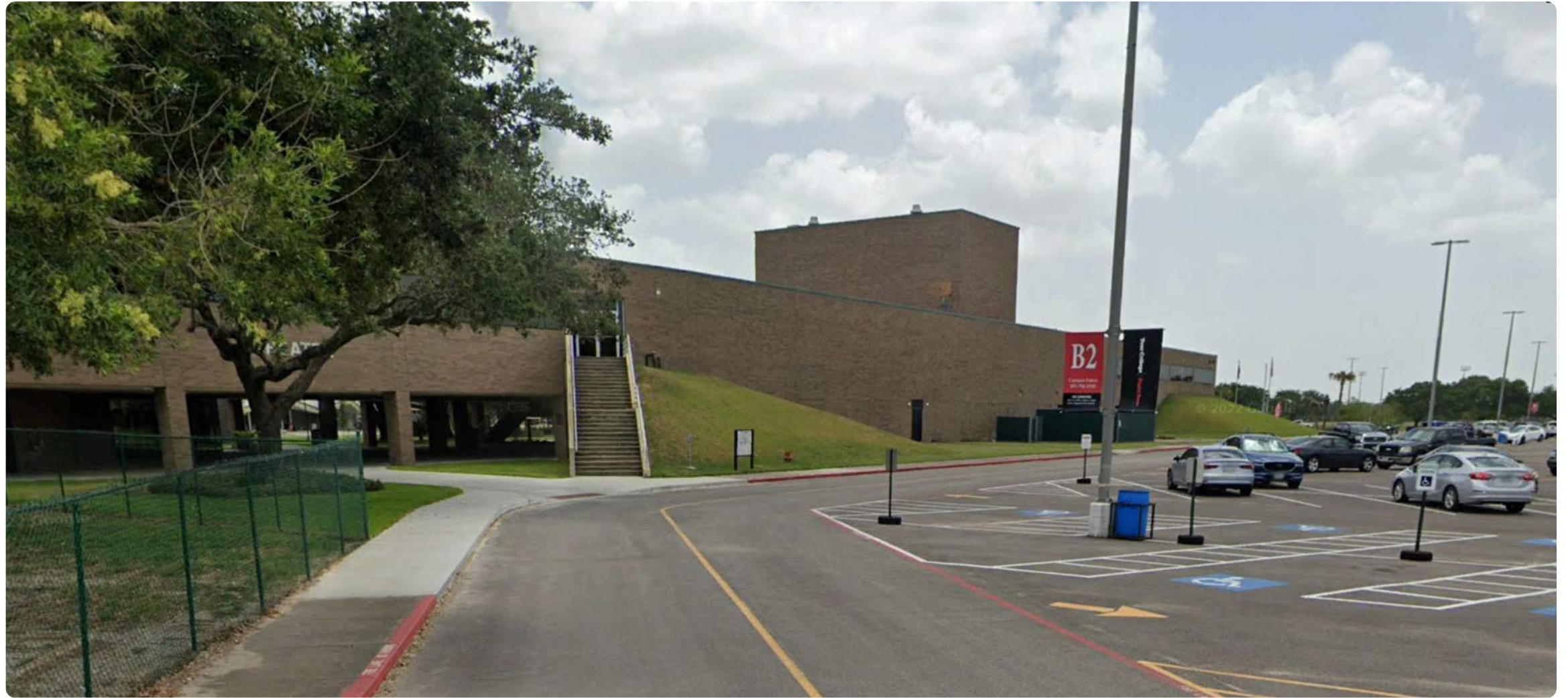
Existing Auditorium Entry
